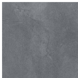
CBC 41522 Kassel Concrete
